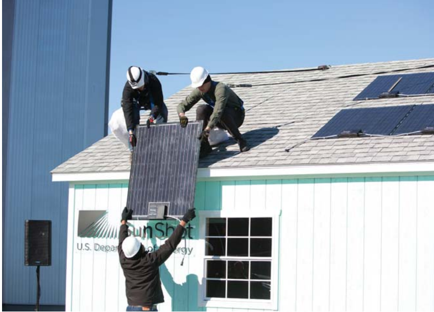
Demonstrating the Installation and Commissioning of Fraunhofer CSE's Plug & Play PV Systems
